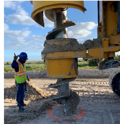
Figure 5: CFA starter during positioning.
