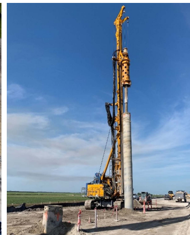
Figure 3: Kelly predrilling and replacement operation.
