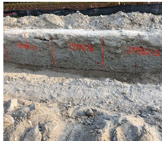
Figure 7: Excavated spoils cutoff wall at TO3.
