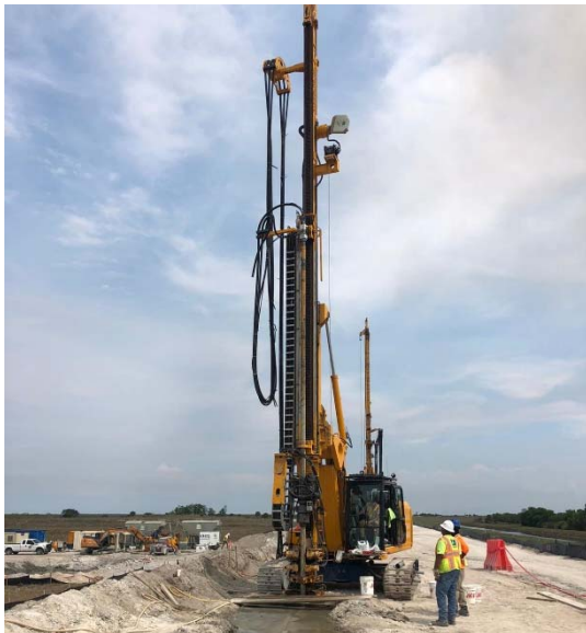
Figure 12: Klemm KR 720 during pre-production trial column installation.
