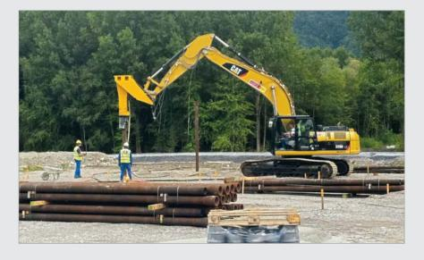
**Chiasso, Aldi, Switzerland** For an Aldi market in Chiasso, Switzerland, 152 nos. ductile piles with 2,250 lin.m were installed by BAUER Spezialtiefbau Schweiz AG for the client Aldi Suisse AG in 2009.
