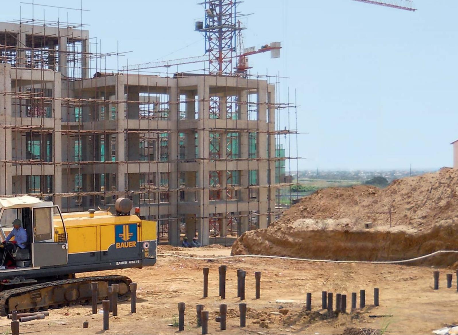
The Bauer DUKI Pile System is a simple, fast and highly effective deep foundation system. The industrially pre-fabricated piles made from high-strength ductile cast iron, guarantee high quality and a safe foundation. To execute the foundation, the individual pile sections are joined together without using special tools to form a pile shaft of any length and vibrated into the soil by a high frequency hydraulic impact hammer. After driving, the DUKI Pile is
