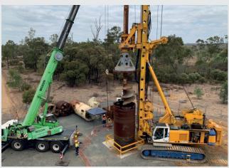
One of our key mining clients in Australia engaged BFA to construct a near vertical ventilation shaft, from the surface, down to the working coal seam below, using conventional piling drill methods. The timeframe and quality of work completed by BFA was extremely valued & recognized by the client and ensured BFA was the market leader for this mining industry requirement.
