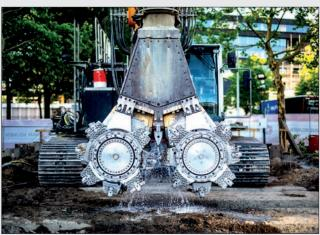
The cutter technique also allows the "hard-in-hard method", whereby secondary panels are cut into the already hardened primary panels.
