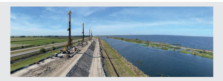
Bauer is proud to have been contracted to execute many cut-off wall projects as part of the Herbert Hoover Dike Rehabilitation in FL, USA. Working both as a General Contractor for the US Army Corps of Engineers or as a Subcontractor. Nearly 28 miles of CSM (over 5 million square feet!) have been installed, starting in 2008 with the Reach 1 task orders, continuing through 2019 with various new culverts and continues into 2022 with the multiple award task orders.
