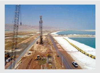
The subsoil presented a special challenge: The hard crystalline salt layers required the use of two Bauer cutter units, in combination with one grab unit. Also, the tremendously critical effect of the high salt content on the support fluid had to be addressed by developing innovative custom-made compositions.
