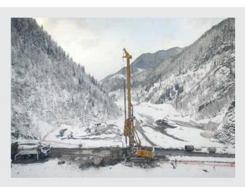
installed as specified, piles at the abutments had to be embedded at least 1 m into the competent rock. Other piles were designed to be embedded into the coarse alluvium, a stratum below a 2 m thick clay layer. All pile depths and rock/alluvium levels were checked and confirmed by inspectors from the Consultant.
