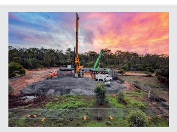
Drilling of 2 m dia through concrete plug and into top of working coal seam roof at 71 m
