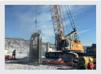
of approx. 3.7 km. The wall had to be embedded into the weak sandstone / mudstone rock. In places up to 3.8 m rock embedment was achieved to reach the designed wall toe levels. The panel excavation reached a maximum installation depth of approx. 25 m.
