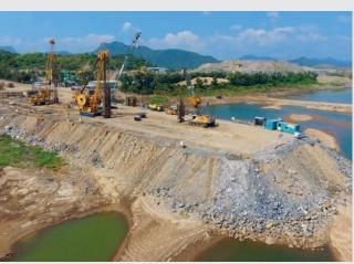
The rivers of the Himalayas have the potential to help achieve the global goals on renewable energy. However, in order to build Hydroelectric Power Plants in the alluvial and colluvial soil formations of these rivers a technology is required to enable cutting through boulder and into the underlying bed rock. With the **Bauer Cutter Technology we have** cut boulder of more than 10 m diameter and bedrock of more than 180 MPa UCS value. This is only possible with **#BAUERPOWER.**
