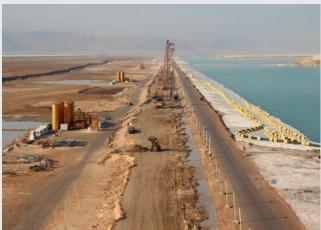
hydraulic head on both sides of the cut-off wall, besides the completely disappeared water flow stretches on the downstream side, provided clear evidence for the success of the executed works to the stakeholders.
