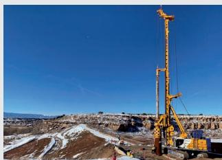
Extract casing with the rotary drive (or alternatively with an oscillator) concurrent with rising concrete level inside the bore.
