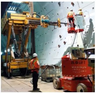
Tunnel under Suez Canal, Ismailia, Egypt Construction of four cross slats to connect two roadway tunnels with brine freezing.
