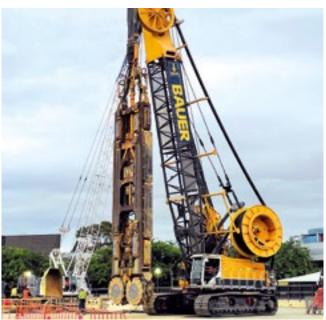
Hobson Bay, Melbourne, Australia Construction of two shafts using an MC 96 duty-cycle crane with a BC 48 trench cutter.
