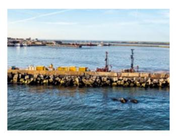
**Southern harbor pier, Helgoland, Germany** By combining mortar with hybrid slurries, 6,307 m<sup>3</sup> of compaction grouting were carried out.
