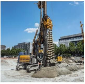
**Parkstadt Schwabing, Munich, Germany**Construction of a 6,000 m<sup>2</sup> single-anchored Mixed-in-Place cutoff wall for a 9 m deep excavation pit.
