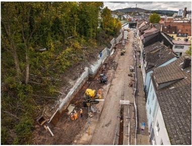
(1) For the expansion of Trippstadter Strasse in Kaiserslautern, Spesa carries out extensive slope safeguarding measures with dismantling and railway embankment reinforcement.
