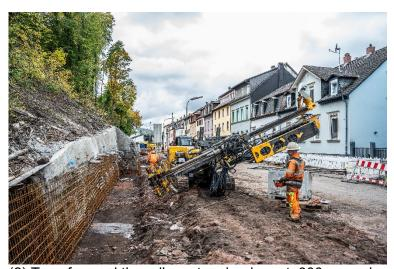
(2) To safeguard the adjacent embankment, 300 ground anchors were installed.
