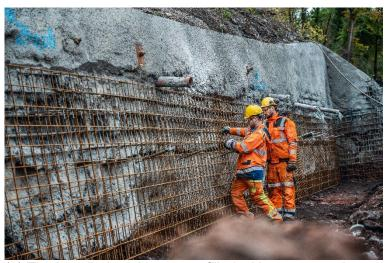
(3) The installed anchors were filled with a cement slurry and further reinforced with welded wire mesh.
