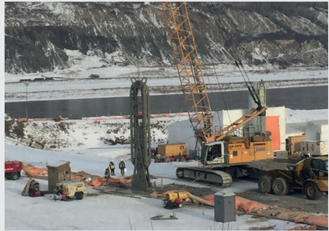
of approx. 3.7 km. The wall had to be embedded into the weak sandstone / mudstone rock. In places up to 3.8 m rock embedment was achieved to reach the designed wall toe levels. The panel excavation reached a maximum installation depth of approx. 25 m.
