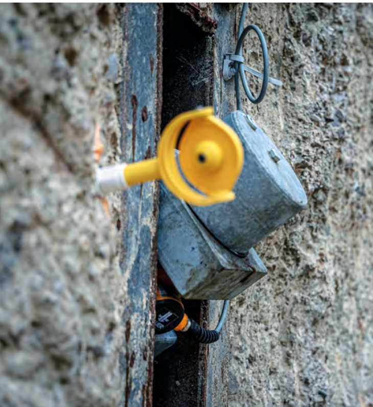
Installed BAUER Load Cell
