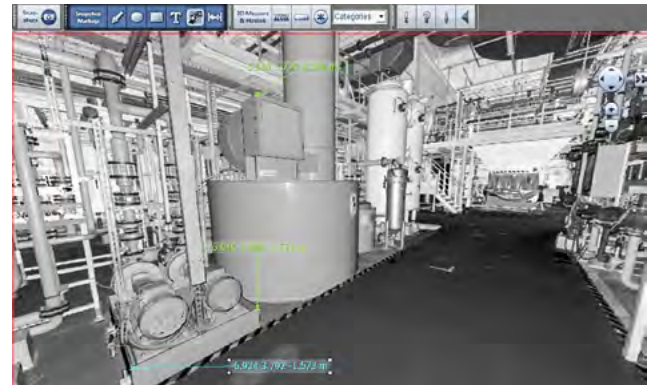
On-site measuring of an existing cleaning plant
