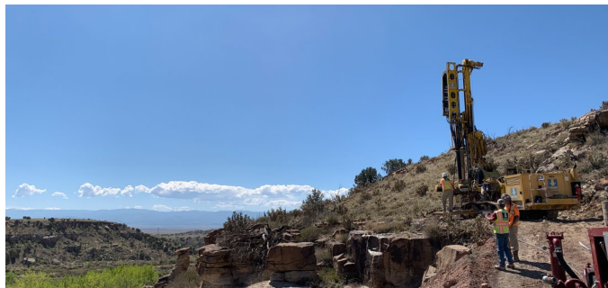
Fig. 17: Grout curtain installation
