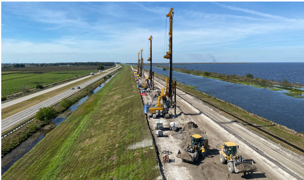
Figure 9: Cut-off wall construction
