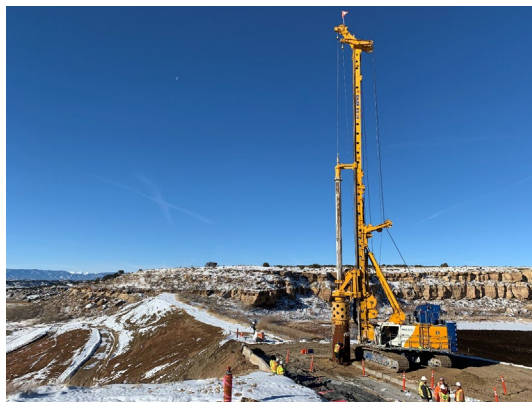
Figure 16: Secant pile wall construction
