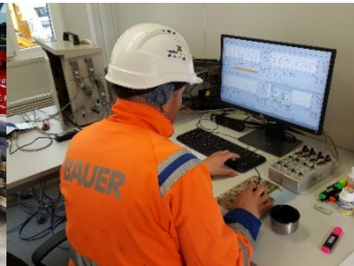
Fig. 6. Controlling and monitoring the grouting work
