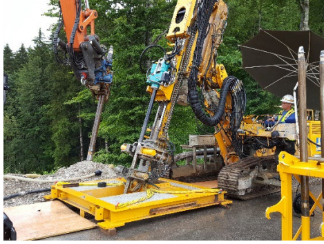
Fig. 3. Drilling inclined holes using KLEMM drill rig
