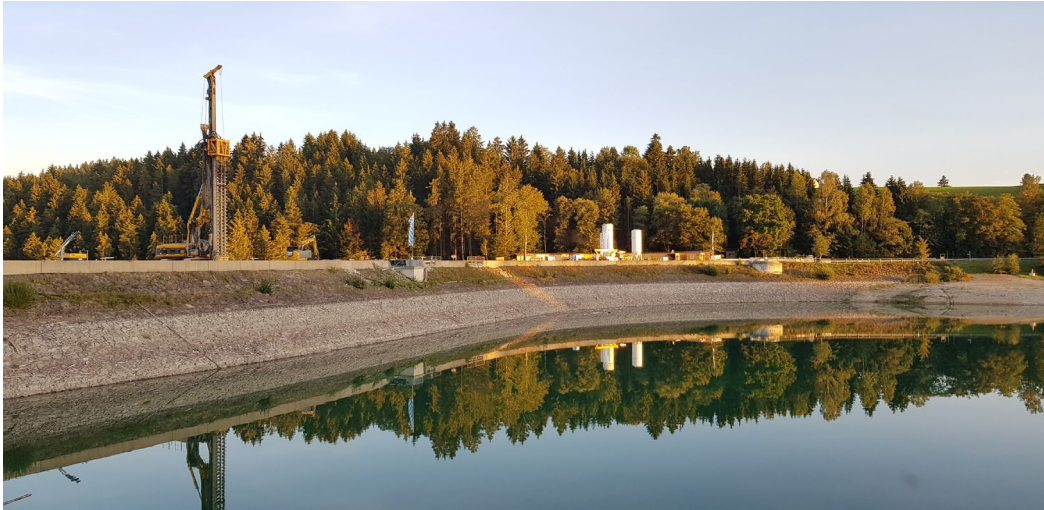
Fig. 8. Execution of the Mixed-in-Place-encasement walls, prior to the diaphragm wall
