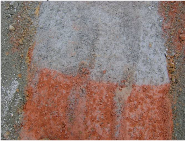
Plate 9 – View of joint between primary and secondary panels
