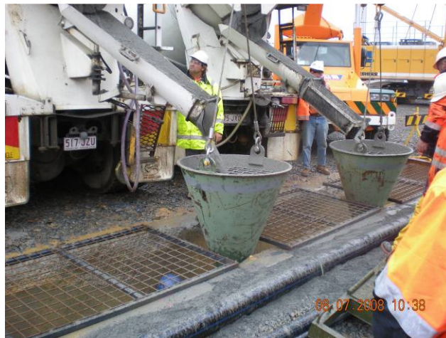
Plate 6 – Concreting of Primary Panels
