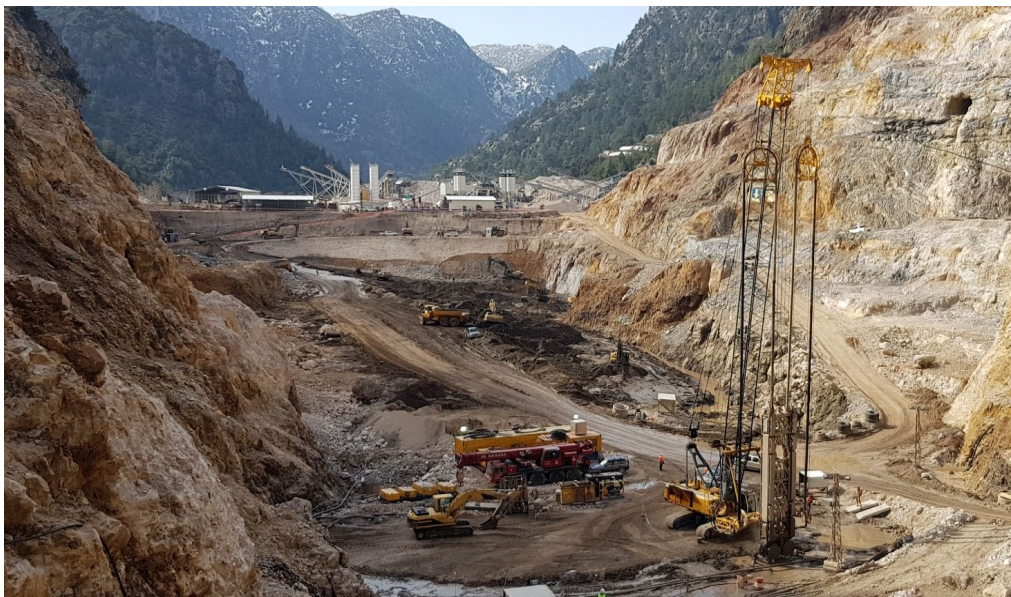
Fig. 11 Execution of diaphragm walls to create a bulkhead
