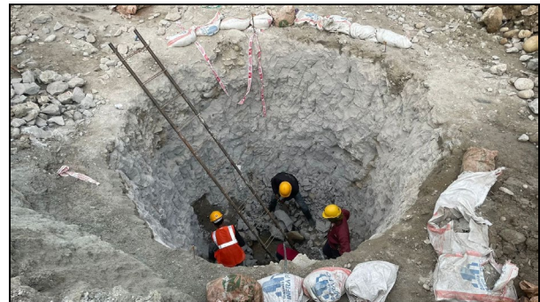
Fig. 5. Excavation of shaft
