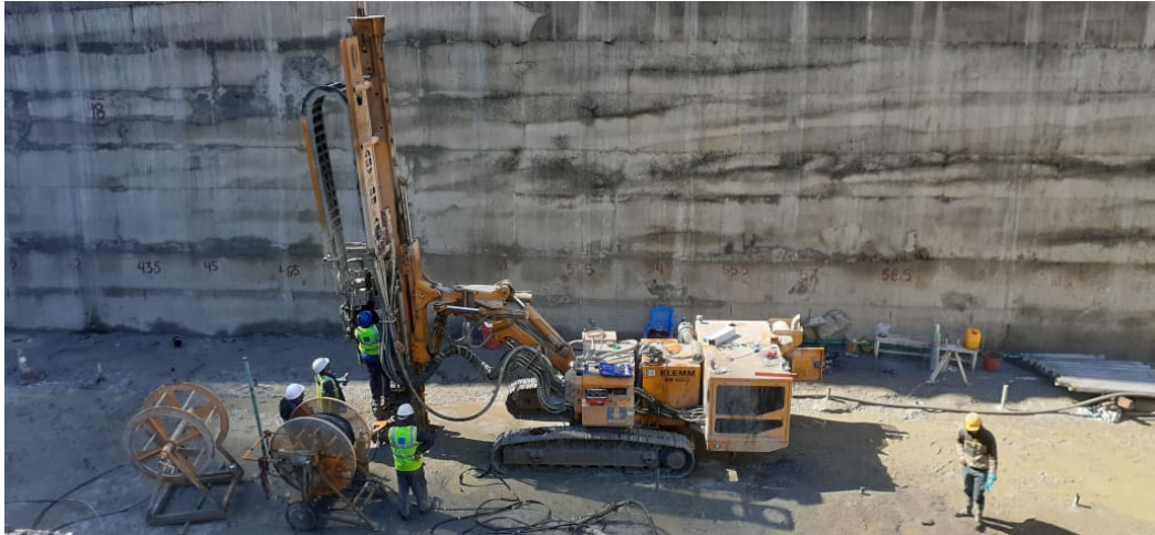
Fig. 8. Drilling and grouting works in progress
