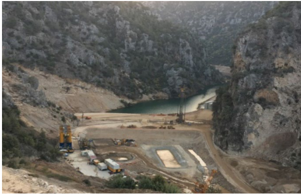
Fig. 3. Execution of cut-off wall at upstream cofferdam
