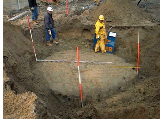
Fig. 5. Jet grout columns with 4.35 m diameter in clean sand
