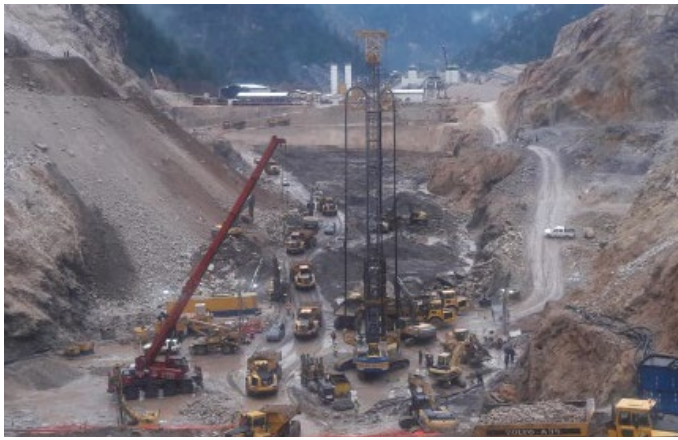
Fig. 13. Imposed congested working zone with dumpers, access road to reservoir, stockpile area through the bulkhead working area
