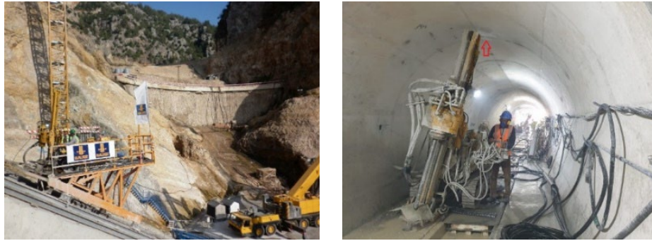
Fig. 14. Mobile platforms for drilling and grouting works on slopes with the exposed bulkhead behind (left) and working in gallery (right)
