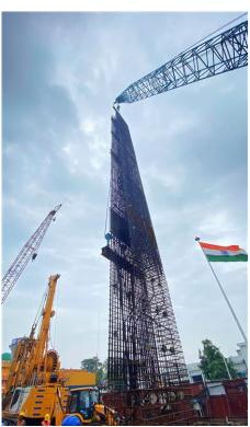
(2) The dimensions of the reinforcement cages are extremely imposing – the deepest diaphragm wall element reached a record depth of 75 m.
