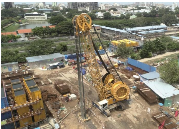
(2) BAUER MC128 duty-cycle crane cutting a panel
