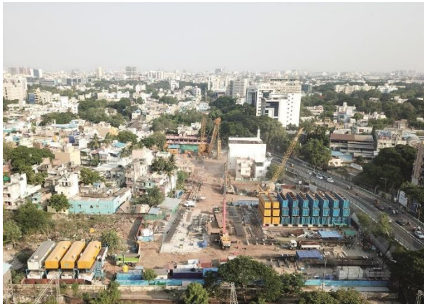
(1) Overview of the construction site in Chetpet, Chennai
