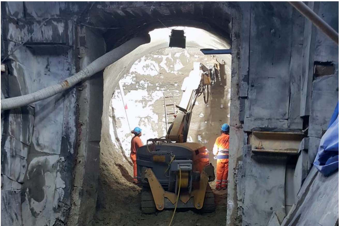
Tunnel Ismailia, excavation of a cross passage
