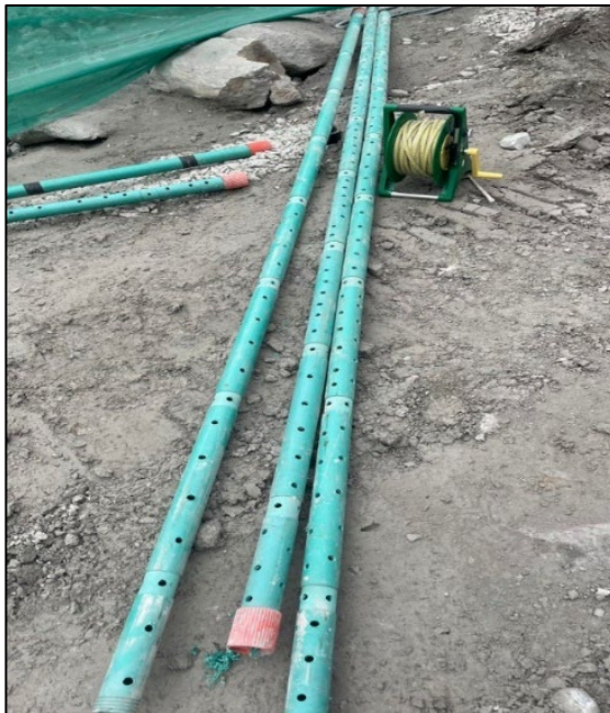
Fig. 3a. Perforated Pipes for Observation Bore Hole
