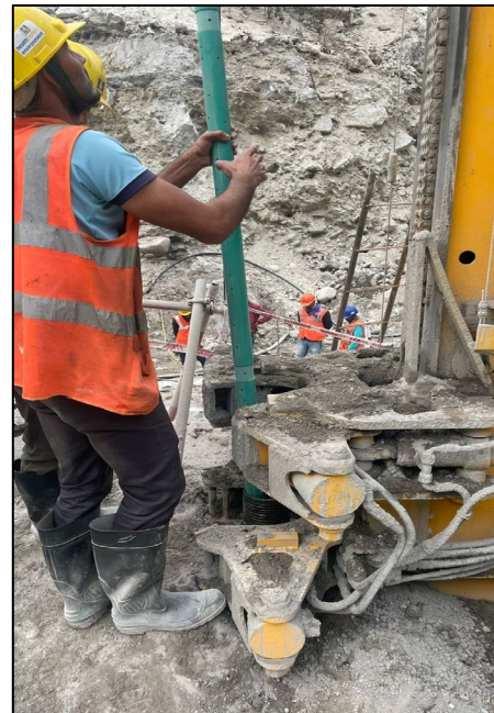
Fig 3b. Installation of perforated pipe
