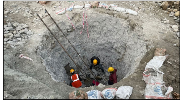
Fig. 2. Excavation of Shaft
