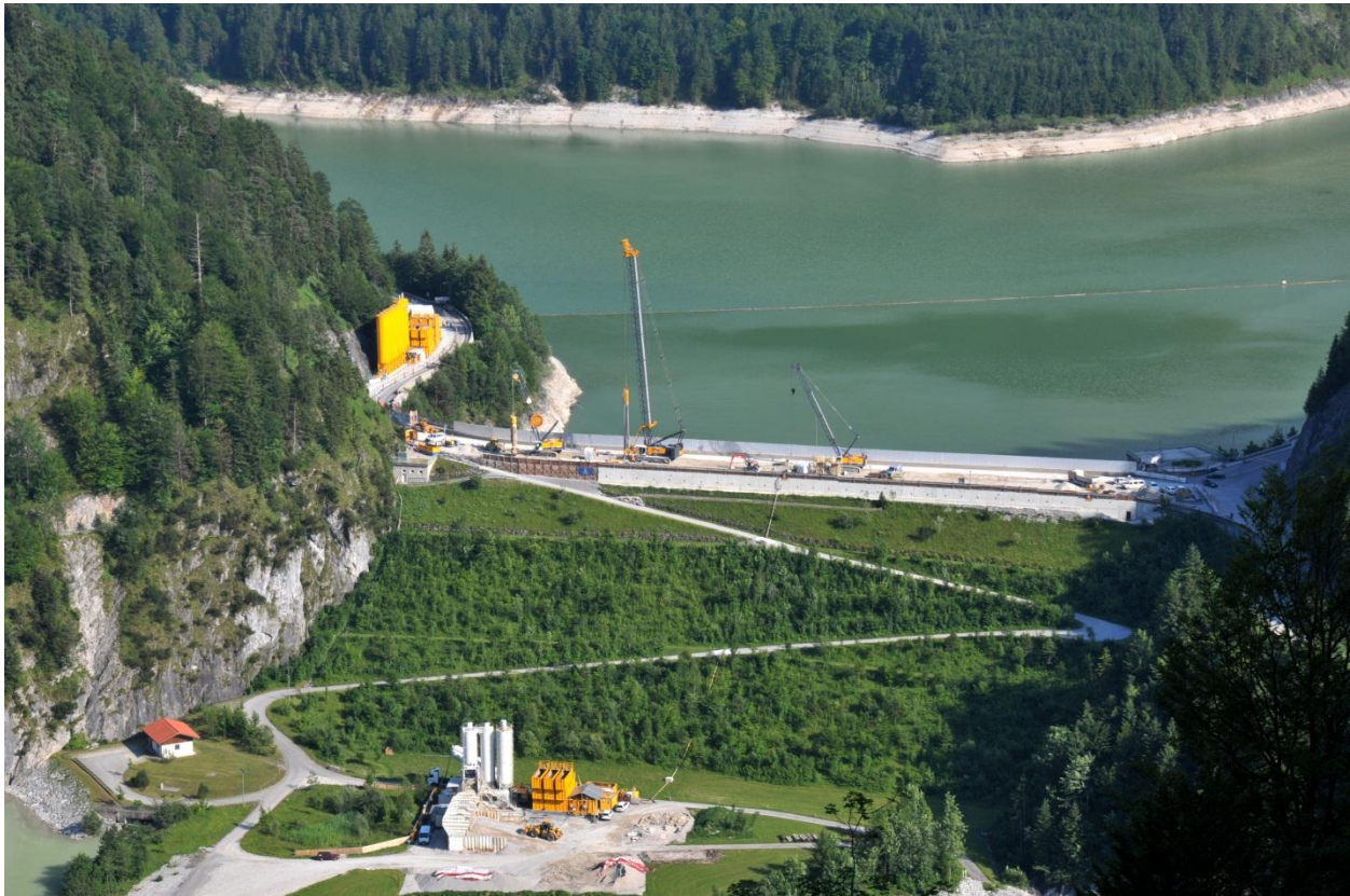
Fig. 3: Sylvenstein Dam – view from downstream – COW under execution.
