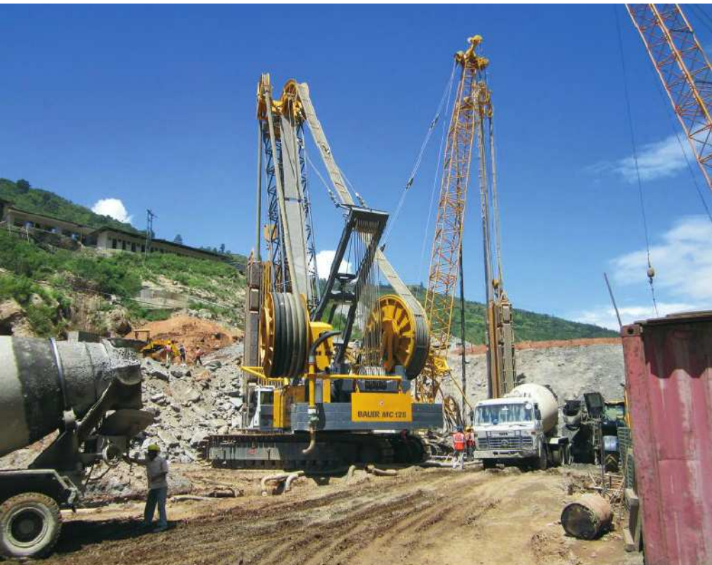
BAUER MC 128 and Trench Cutter BC 40 (© BAUER)
