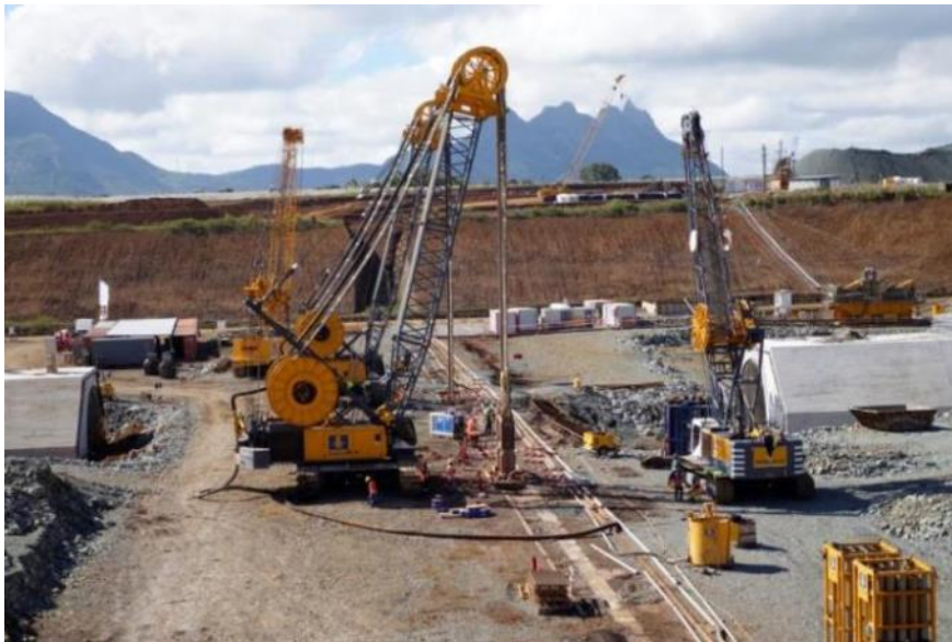
Figure 1 BAUER Trench-Cutter and Grabs along the CCOW installation
